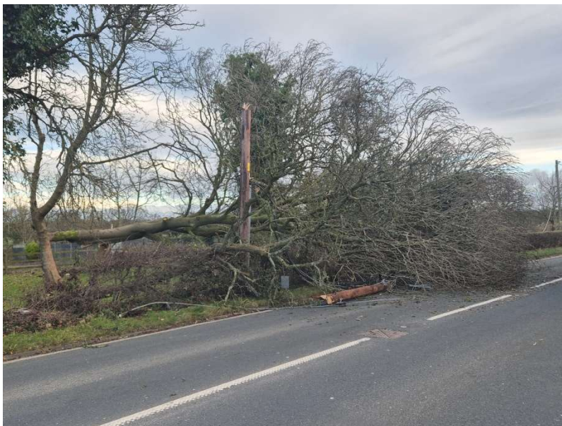
A snapped pole can be seen underneath this fallen tree during Storm Darragh – December 2024.
