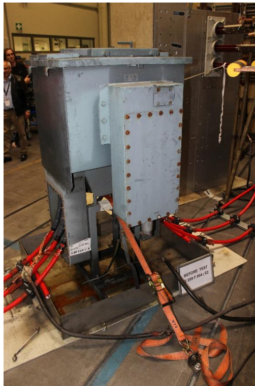
Photo No. 02: Before test XZ 289 F 004 / 02 Test object, rear view
