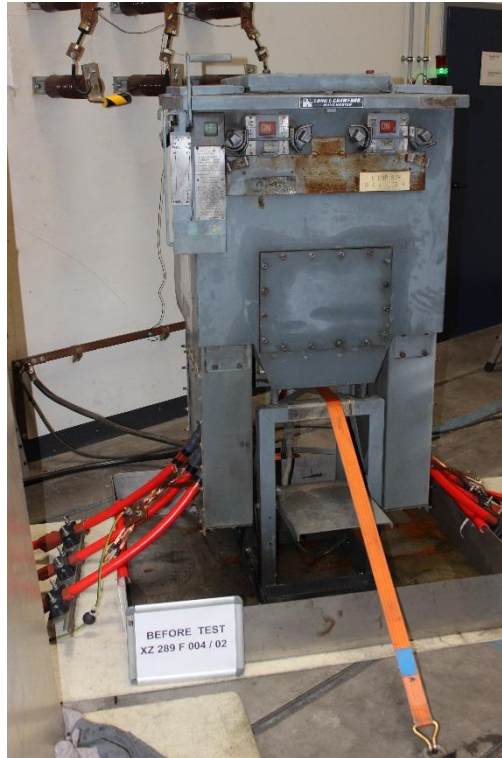
Photo No. 01: Before test XZ 289 F 004 / 02 Test object, front view
