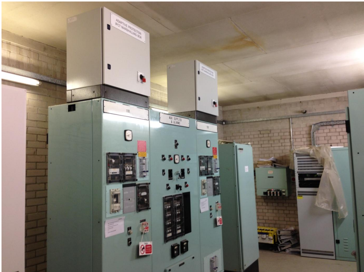
Photograph 2: Type 1 installation showing Interposing Current Transformers (IPCT) boxes mounted on top of T11 and T12 11kV Protection panels at Irlam Primary.
