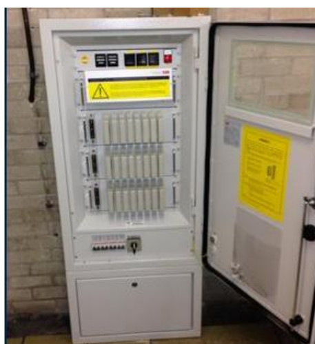
Figure 3.14: I_S sensing unit at Wigan BSP
