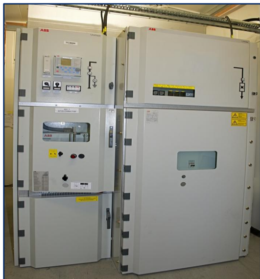
Figure 3.11: Broadheath I_S -limiter and series CB
