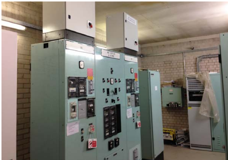
Figure 2a: Adaptive protection relay fitted in existing panel at Blackbull
