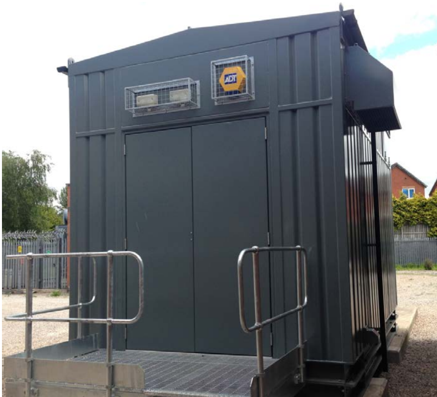
Figure 5a: I_S Limiter container at Bamber Bridge
