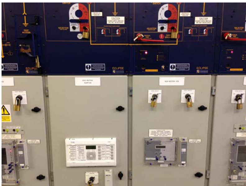
Figure 2a: Adaptive protection relay fitted in existing panel at Blackbull
