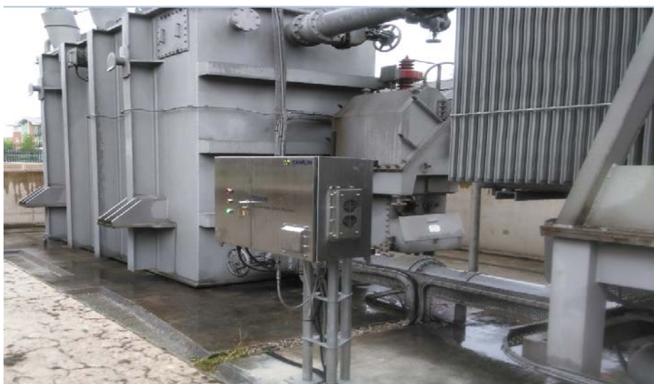
Figure 12: Kelvatek TOTUS dissolved gas analysis installation
