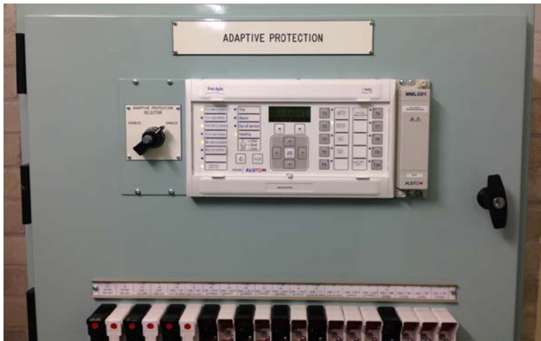
Figure 1: Irlam 6.6kV Adaptive Protection
