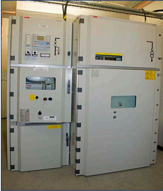
Figure 5a: I_S Limiter container at Bamber Bridge
