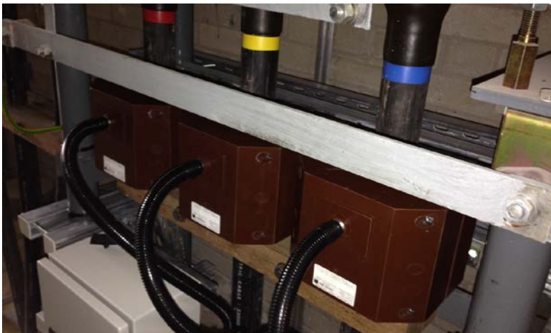
Figure 5e: IS sensing unit CT data plate at Wigan on the Gidlow No1 33kV circuit
