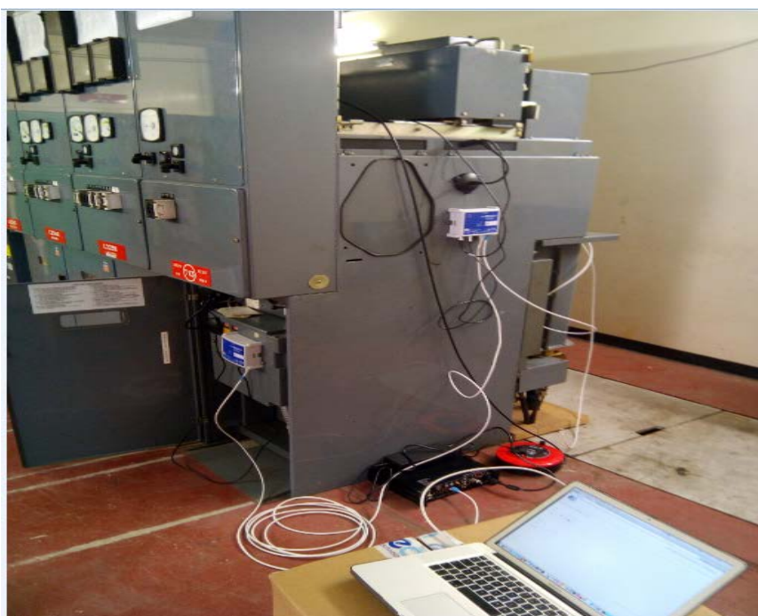
Figure 10: EATL Ultratev installation at Broadheath
