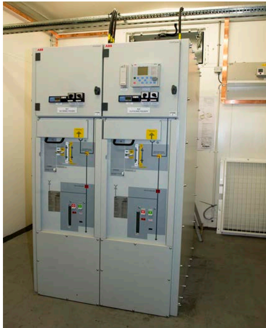
Figure 5: Broadheath I_S -limiter bypass
