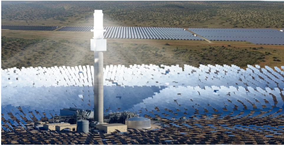
FIGURE 7: CSP MOLTEN SALT SYSTEM, WITH RECEIVER TAKING CONCENTRATED SOLAR BEAMS REFLECTED BY HELIOSTATS. [6]
