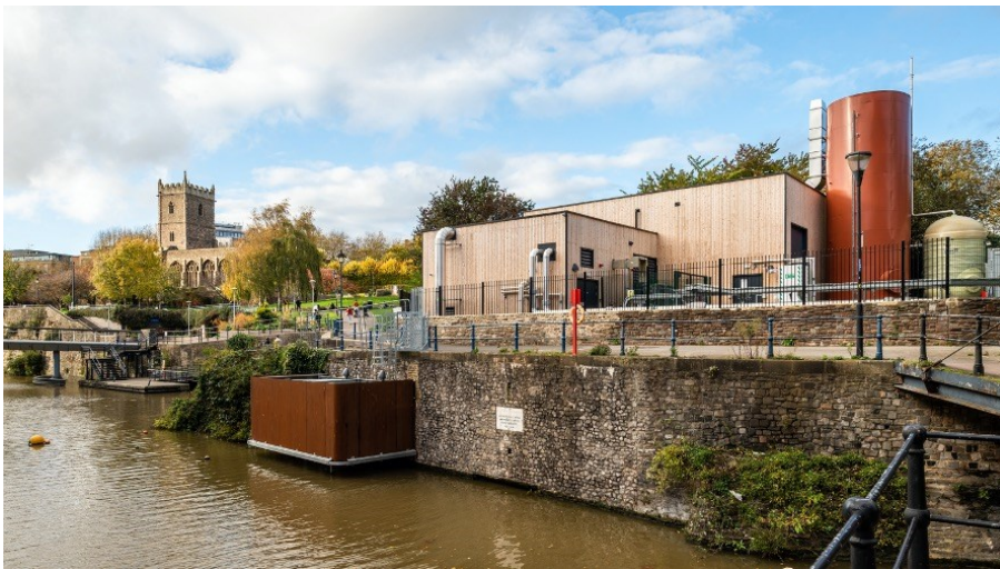
FIGURE 10: 3MW WATER HEAT PUMP AT CASTLE PARK IN BRISTOL, USED FOR DISTRICT HEATING [9]
