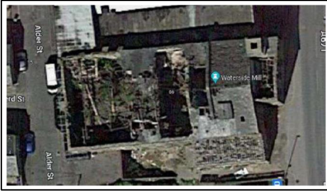
Figure 7-4 Waterside Mill - Roof in need of repair
