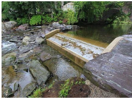
Coanda screen and intake
