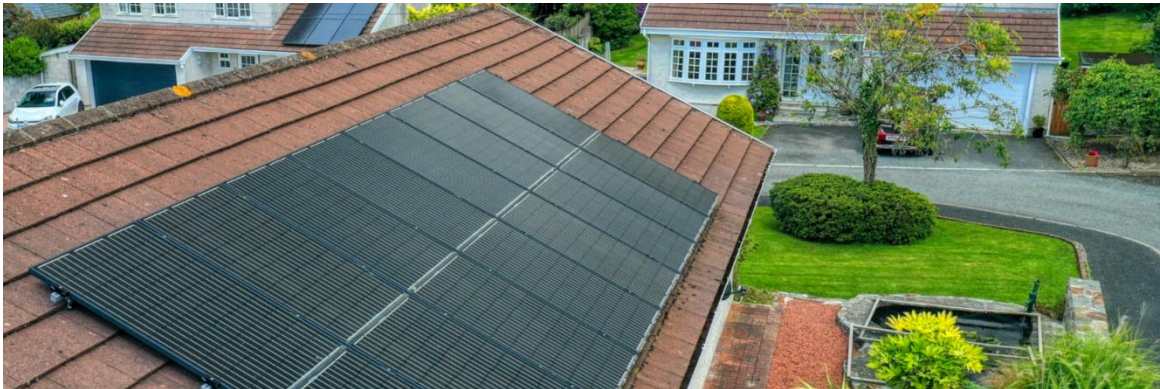
Figure 2-3 - Rooftop mounted PV system example
