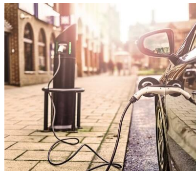
Figure 2-16 Example standard in-street EV charger
